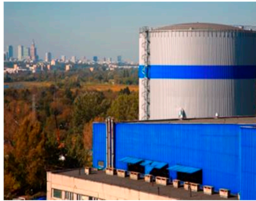
Figure 2. View of the TES tank in Warsaw CHP plant Siekierki.
